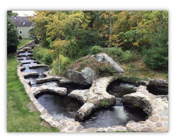
The recently renovated fish ladder rises 42 vertical feet, with 69 pools connected by short waterfalls the fish must scale. LAUREL AMES
